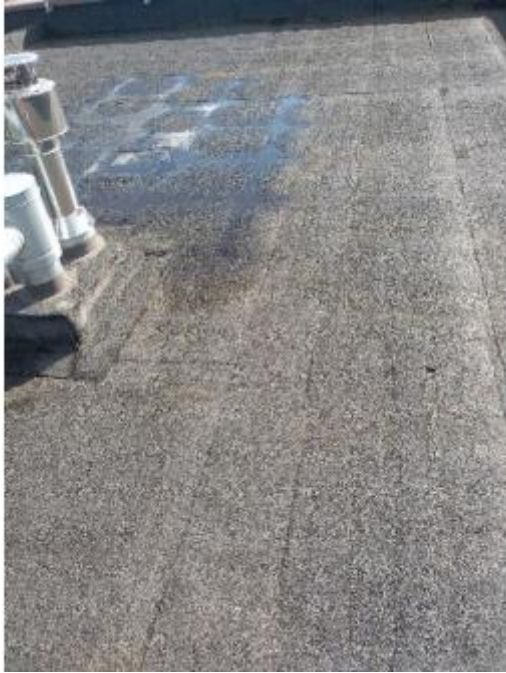
Photos points singuliers crosse, ventilation, lanterneau...
