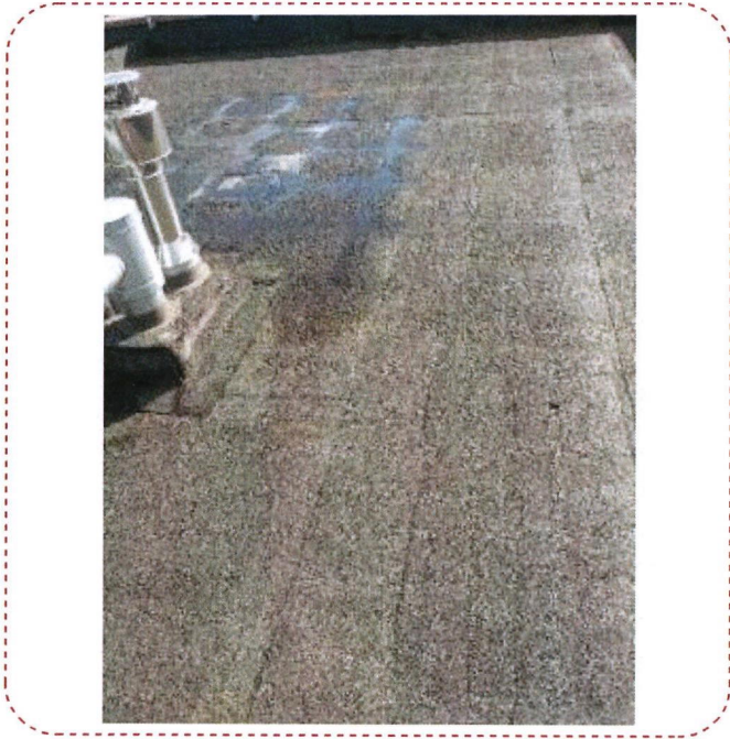
Photos points singuliers crosse, ventilation, lanterneau...
